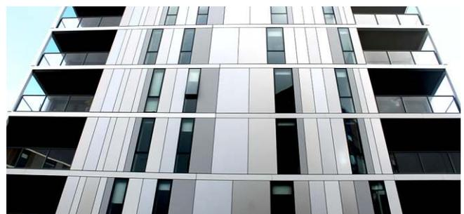
**larcore**® for use on outdoor façades must be installed with the **HideTech**® **Plus** system certified with ETE / ETA (double edging and perimeter riveting) or with system for watertight panel solution.
