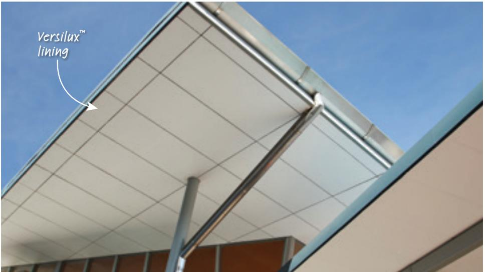
6mm Versilux™ lining with James Hardie™ Black PVC Eave and Soffit Joiner for an express joint look.
