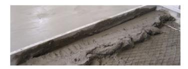
Emaco® Nanocrete R2 is a non-structural re-profiling mortar that is fast setting and suitable for repairs from 3mm to 100mm. Its low resistivity formulation makes it an ideal mortar for bedding passive and discrete anode systems.
