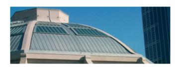
Masterseal® 150E (Barracryl Elastic) and Masterseal® 160D (Barracryl D) anti-carbonation coatings for concrete structures are available in a range of designer colours to suit a wide variety of architectural design needs.
