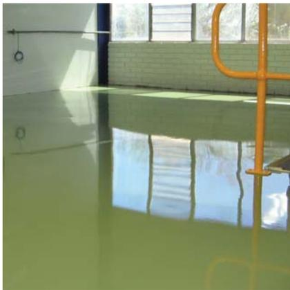
These coatings can be applied in a number of textures to give extra slip resistance in wet areas or to provide improved slip resistance for forklifts. As the aggressiveness of the environment increases, so then does the thickness of the floor from less than 1/2 mm to 2-3 mm for longer lasting and harder wearing floors. These toppings can also be
