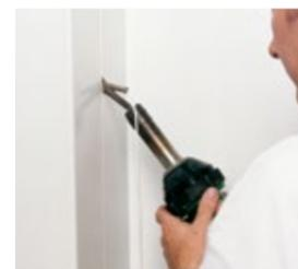
For the highest level of hygiene Altro Whiterock can be fitted using welded joints
