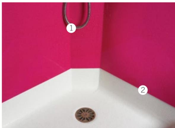
1. Thermoformed corners that are smooth and easy to clean, with no crevices that harbour bacteria
