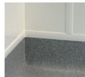
Sealed hygienic environments: through the use of Altro Whiterock FlexiJoint, 2-part jointing system or transition strips
