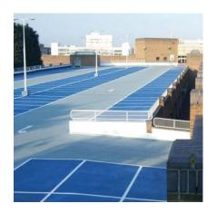
Conipur® fast cure range of primers, membranes, wearcoats and topcoats which allow the complete reinstatement of the full system and return to traffic after only 12 hours.
