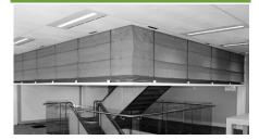
Open up stairwells or protect escalators by using Vertical or Concertina fire and smoke curtains. The Concertina product has been used to fully encapsulate stairs or escalators to allow open plan designs, without the need for columns or walls.
