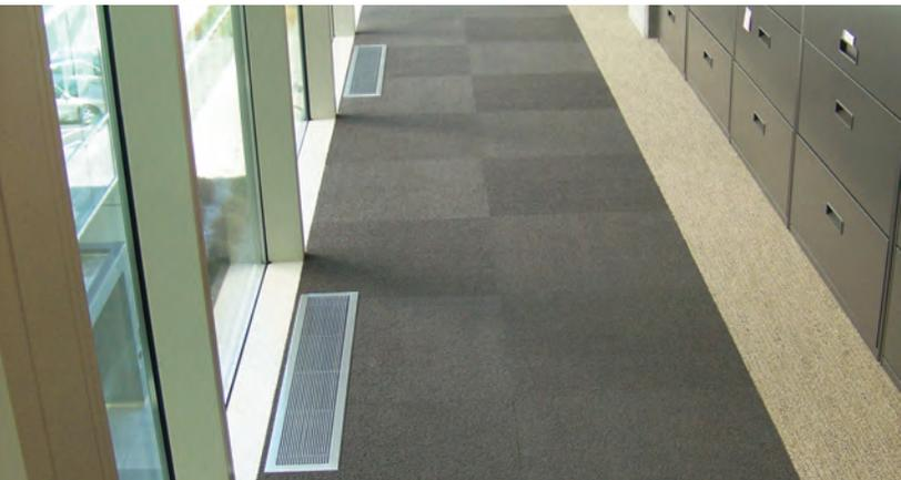
Segmented In-floor Active Chilled Beam application
