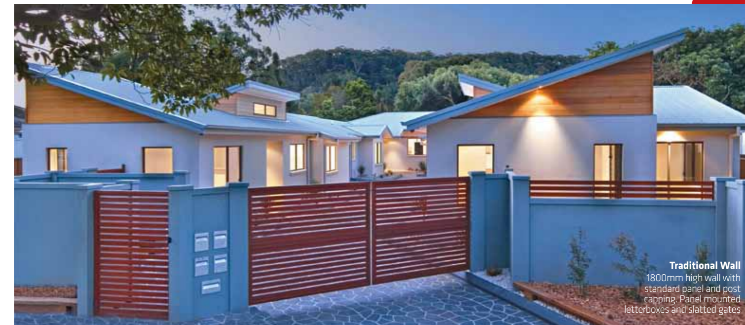
Traditional Wall 1800mm high wall with flush panel and post capping. Post mounted lighting and stone feature
