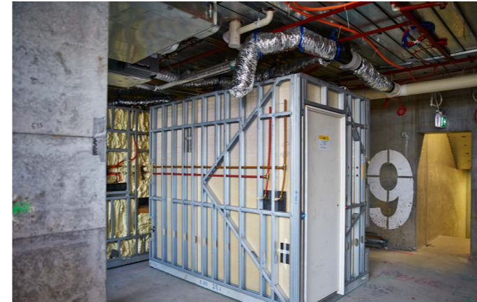
5. POD PLACED AND UNWRAPPED
