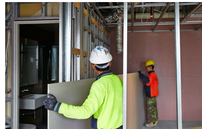
8. EXTERIOR SHEETED WITH PLASTERBOARD
