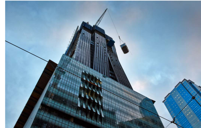
2. POD LIFTED VIA CRANE
