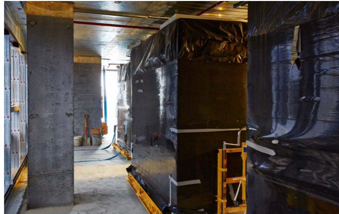
4. POD MOVED INTO POSITION VIA TROLLEY
