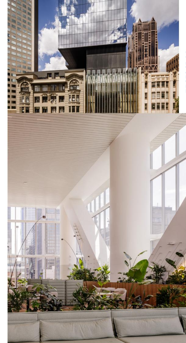
The project's steel mega-column and truss centered design enabled a cantilever to be constructed over the adjoining Heritage building, which allowed larger floor sizes above.
