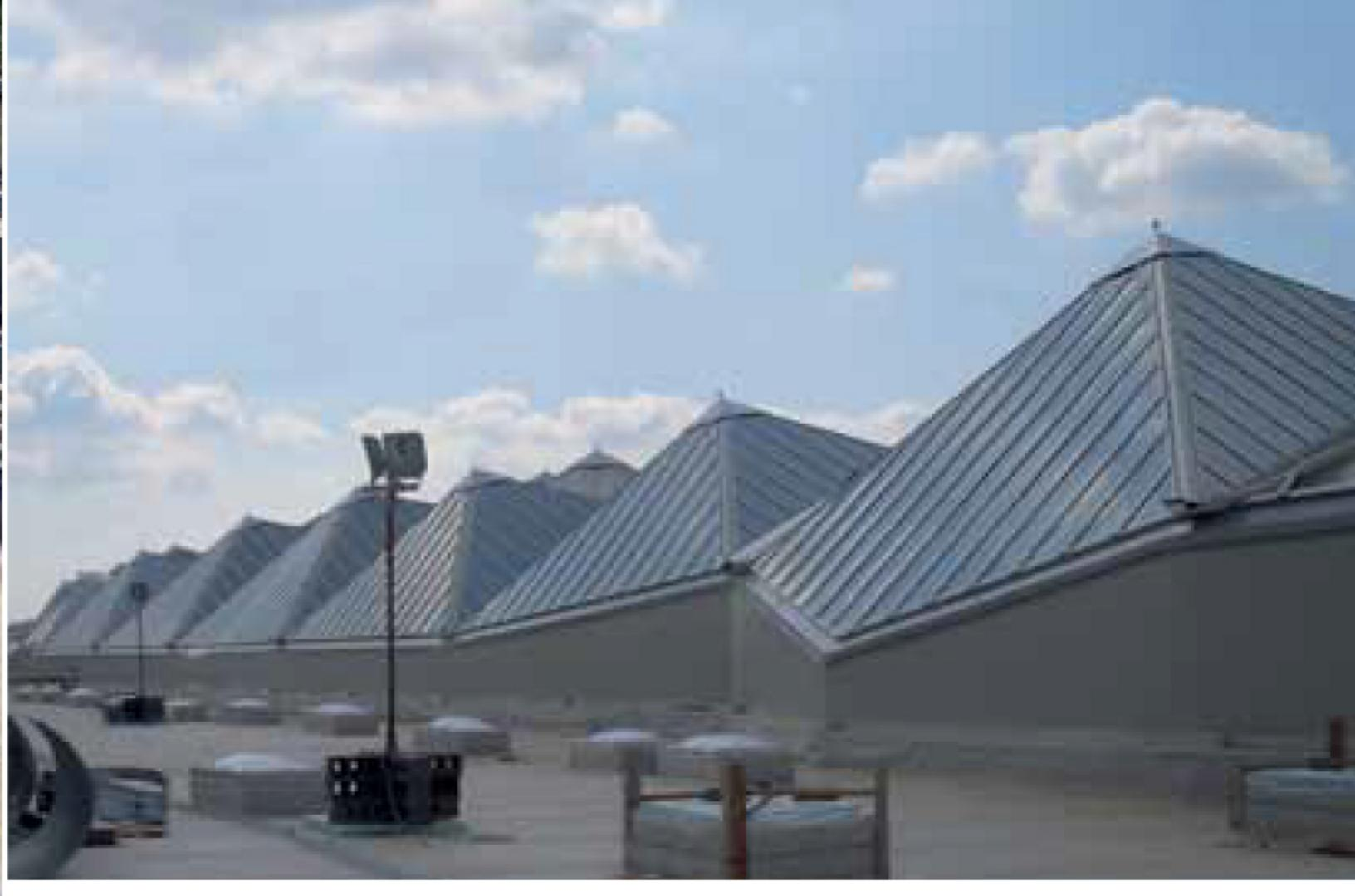
The solution chosen was to connect the upper translucent surface with the steelwork below using short tubular legs, so the two structures are close enough to give the desired effect. The solution used is a complete and tested "roof system". An exclusive system including aluminum profiles, with special joint and adjustable brackets, specifically designed by the company Lazzaro Srl.
