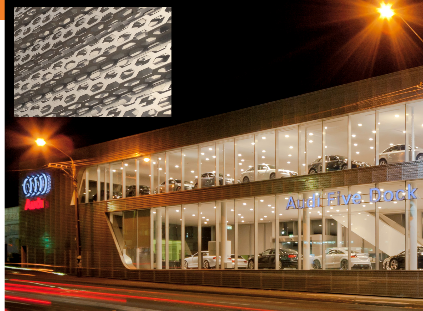
▲ The Five Dock, Sydney, Audi "Terminal" constructed in 2008 was the world's first in this design. The long term durability of the edge surfaces is paramount to maintain the brilliance and metallic lustre of the façade. Anodised in AAF Evershield "Diamond Light". (Disclaimer: Not all Audi terminals are anodised by AAF).
