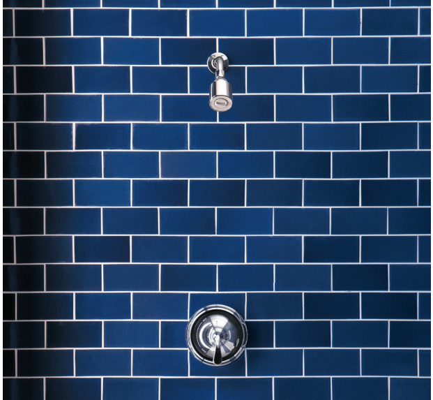
ABOVE: Existing showerhead and mixer, before installing HydroRail using the same plumbing.
