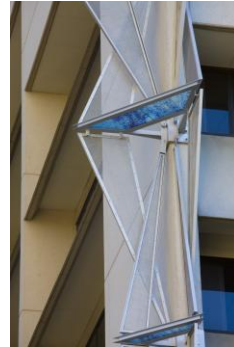
* Typical Architectural Installation
