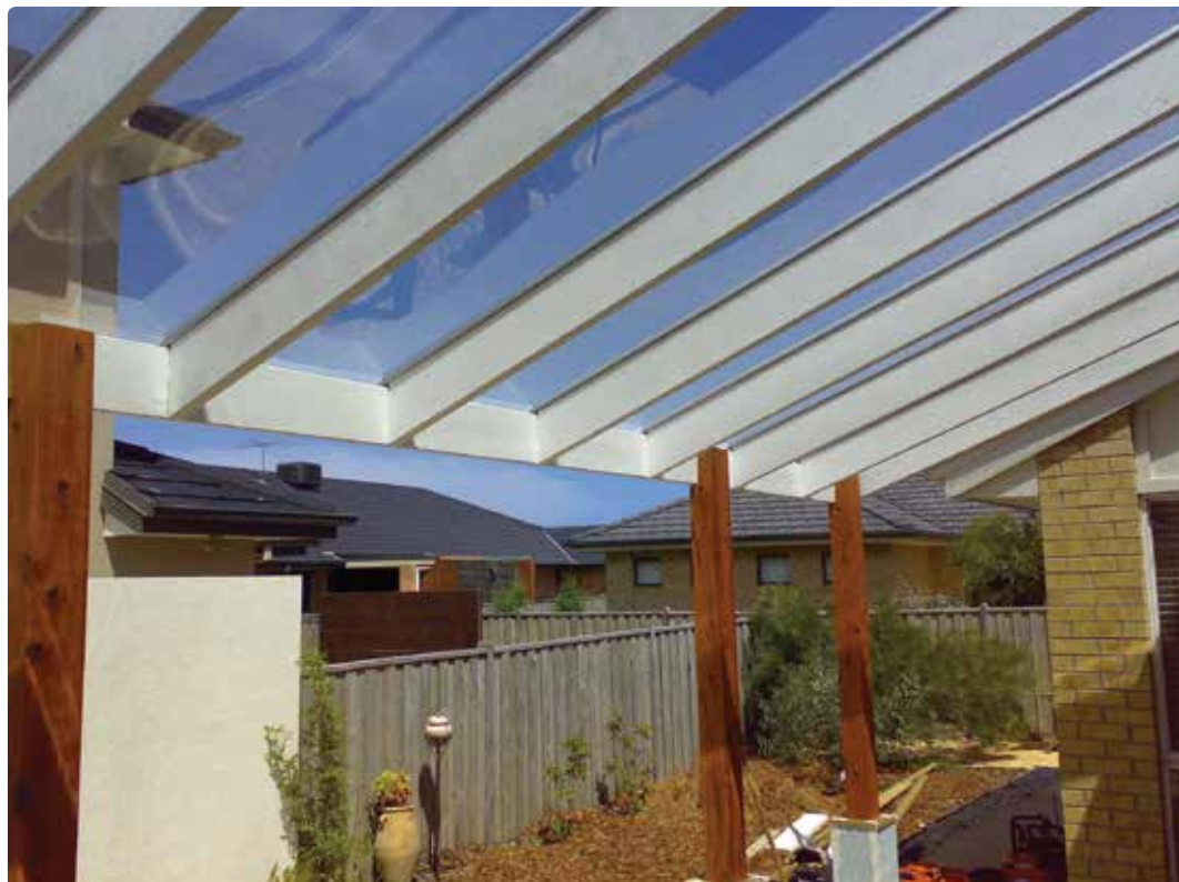
Project: Private home, Point Cook, Australia | Application: Pergola | SUNGLAZE™ Type: Clear 3mm
