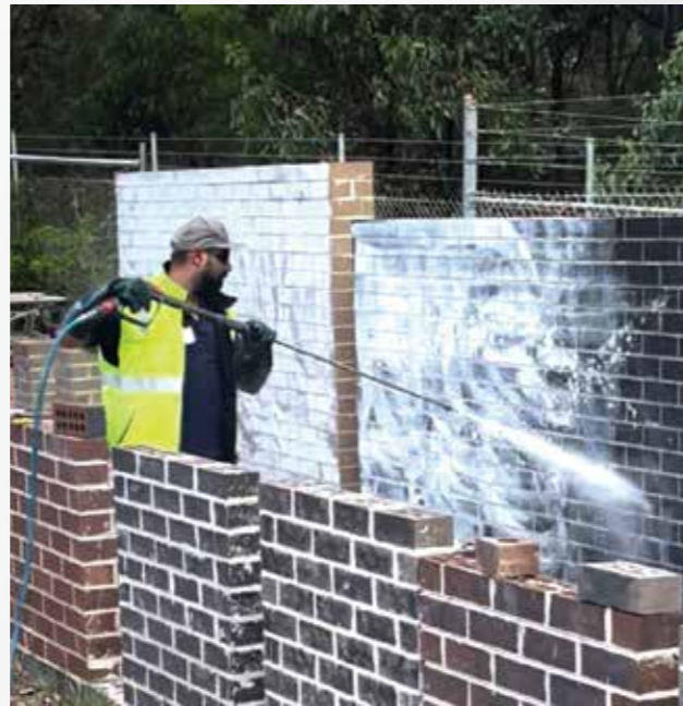
Image: High pressure water cleaning.
