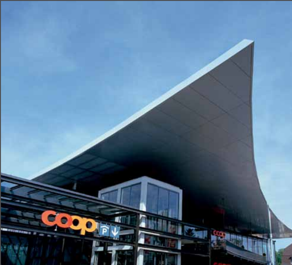
Stable – large, self-supporting roof with ALUCORE® cladding
