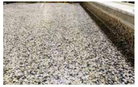
Steel platform, Cowra Abattoir
