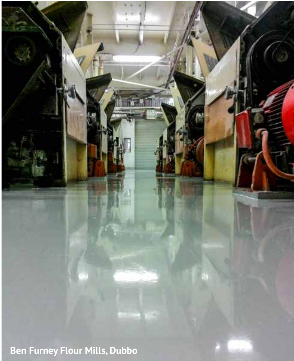
Flooring refurbishment in B61 Harbour Blue
