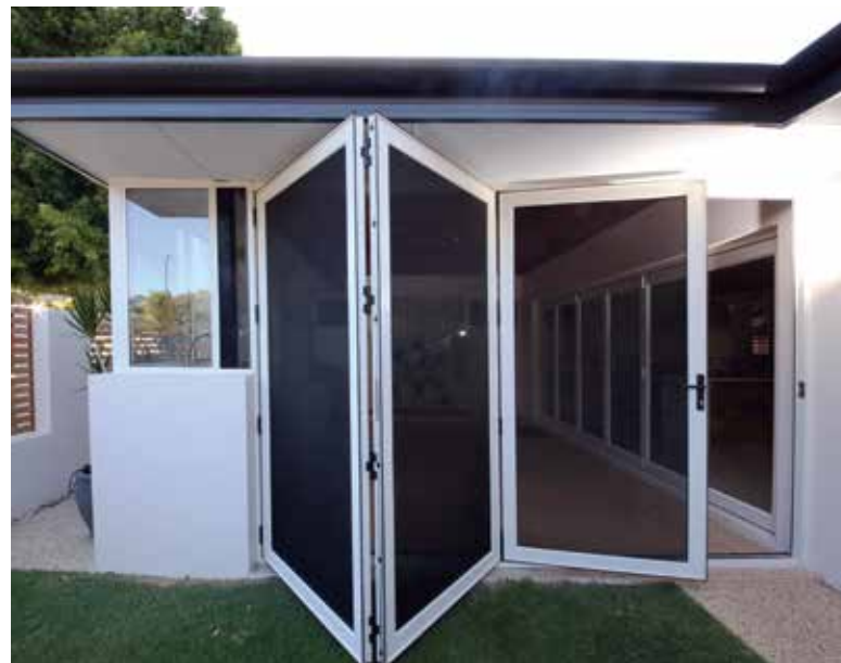
Bi-fold doors are hinged and can fold back to completely open up a living space.
