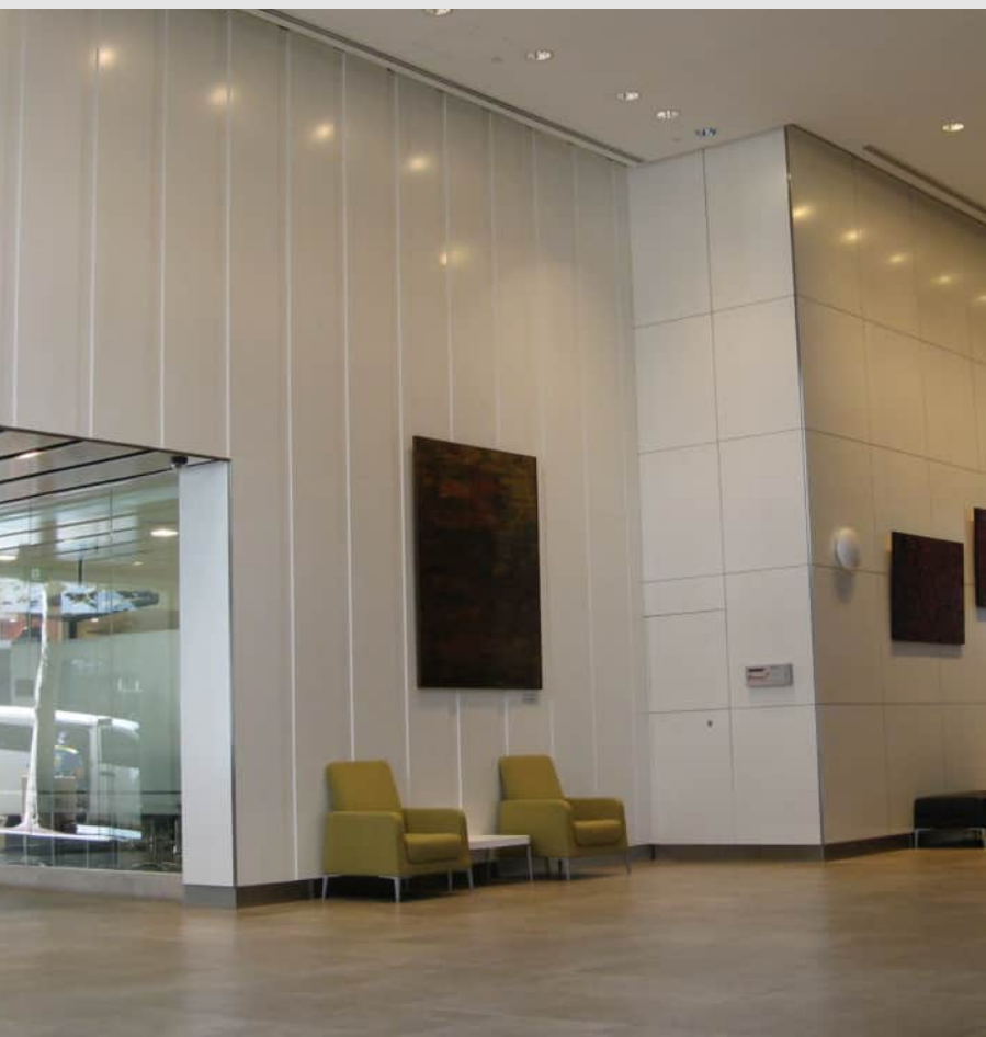
▼ SUPACOLOUR panels form a durable and attractive entry to a city building with extra wide joints and matching backing strips.
