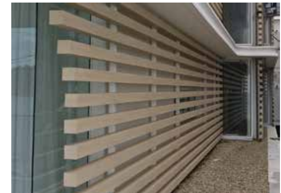
Kabebari 100 x 100 @ 200mm centres | Oku
