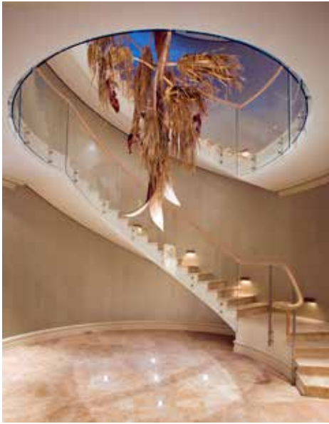
12mm starphire low iron toughened curved glass. Frameless side fix standoff fittings timber handrail capping to top edge of glass
