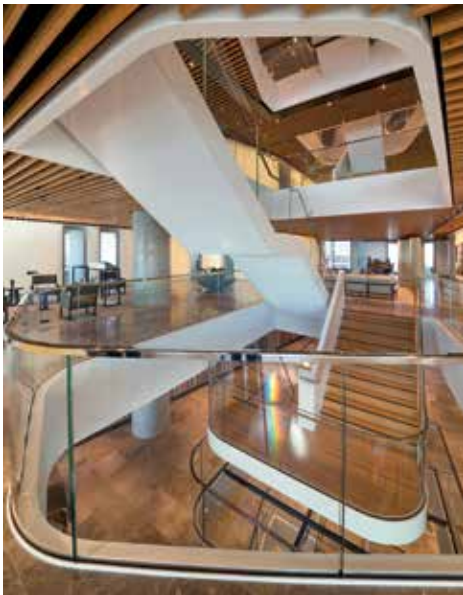
21.52mm Low iron toughened laminated curved glass void balustrade
