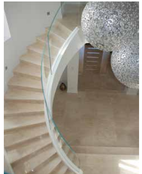
15.04mm Starphire toughened structural laminated curved glass stair balustrade. Engineered glass fully frameless without top rail
