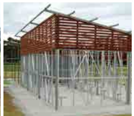
STEEL FRAMEWORK AND WALLS ON-SLAB
