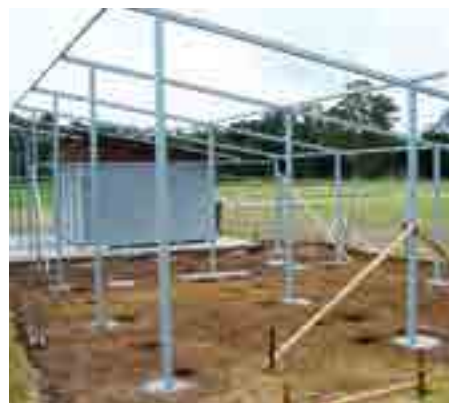
STEEL FRAMEWORK WITH FOOTINGS
