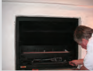
Burner inserted and connected to fixed gas line.
