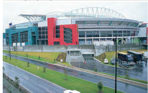
Colonial Stadium – Melbourne
