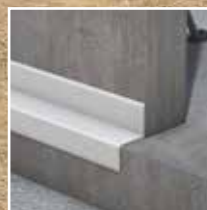
Connection joint between of precast elements
