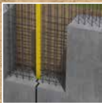
Connection joint with aof diaphragm wall
