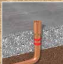
Sealing of penetrations
