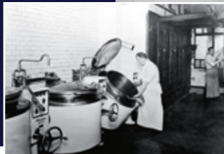
First generation of tilting boiling pans 1934
