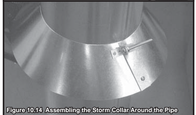
Figure 10.13 Assembling the Storm Collar
