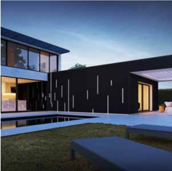
Filled with LED modules
