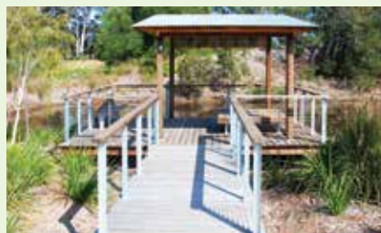
K1162 VIEWING PLATFORMS
