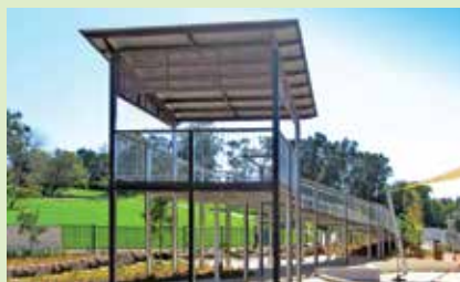
K1172 VIEWING PLATFORMS
