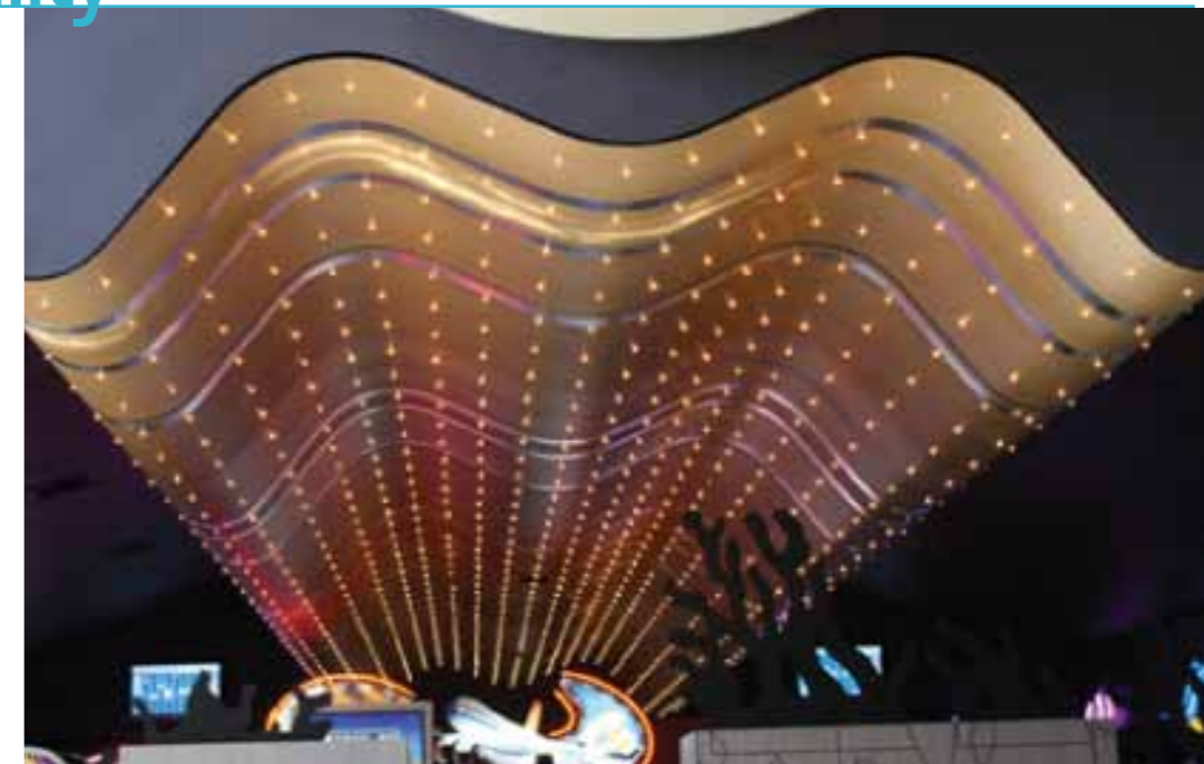
DI-NOC Fine Wood and Metallic are flexible enough to be applied to an existing bulkhead to give the illusion of density without the weight. Courtesy Redcliffe RSL, Qld and Brand + Slater Architects
