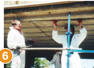
3 Apply MBrace Laminate Adhesive to substrate
