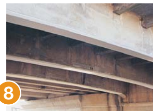
6 Position MBrace Laminate and apply to substrate
