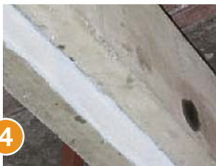
4 Levelling of surface with MBrace Laminate Adhesive
