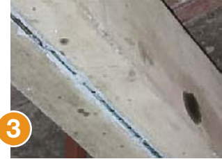
3 Placing Mbar
