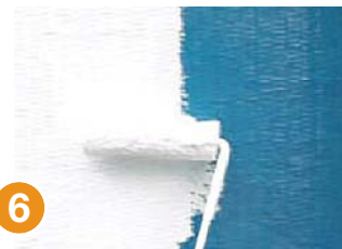
3 Apply first coat of MBrace Saturant
