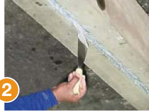
2 Apply MBrace Primer (optional) followed by MBrace Laminate Adhesive onto groove
