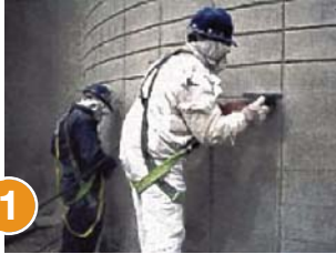
1 Grooving the surface of the concrete
