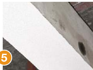
5 Apply MBrace Topcoat (optional)
