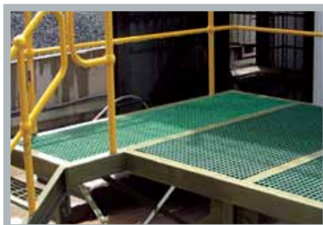
Concrete batching plant, Busselton, WA
