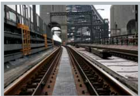
Sydney Harbour Bridge rail walkway
