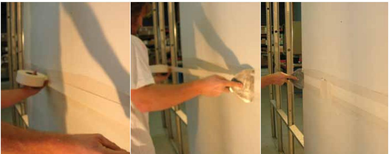
Fill joint with single, thin layer of plaster and then overlay reinforcing mesh.
