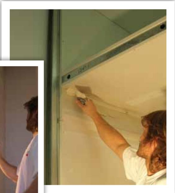
Plastering the board joints in partitions (left) and the junctions of wall and ceiling (above).
