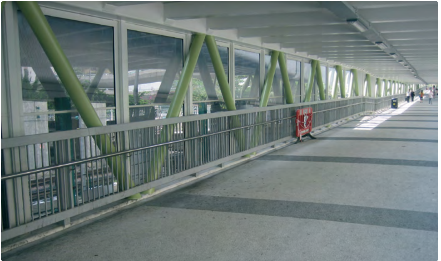
Project: Kowloon Bay MTR (Metro Station) - Hong Kong, China (2008) | Barrier Glazing: PALGLAS® 20mm Grey
