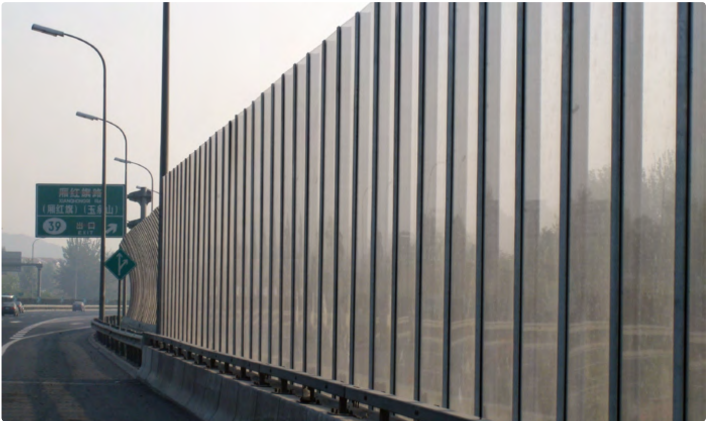
Project: Beijing Ring Road 6 - China (2006) | Barrier Glazing: PALSUN® 6mm Clear
