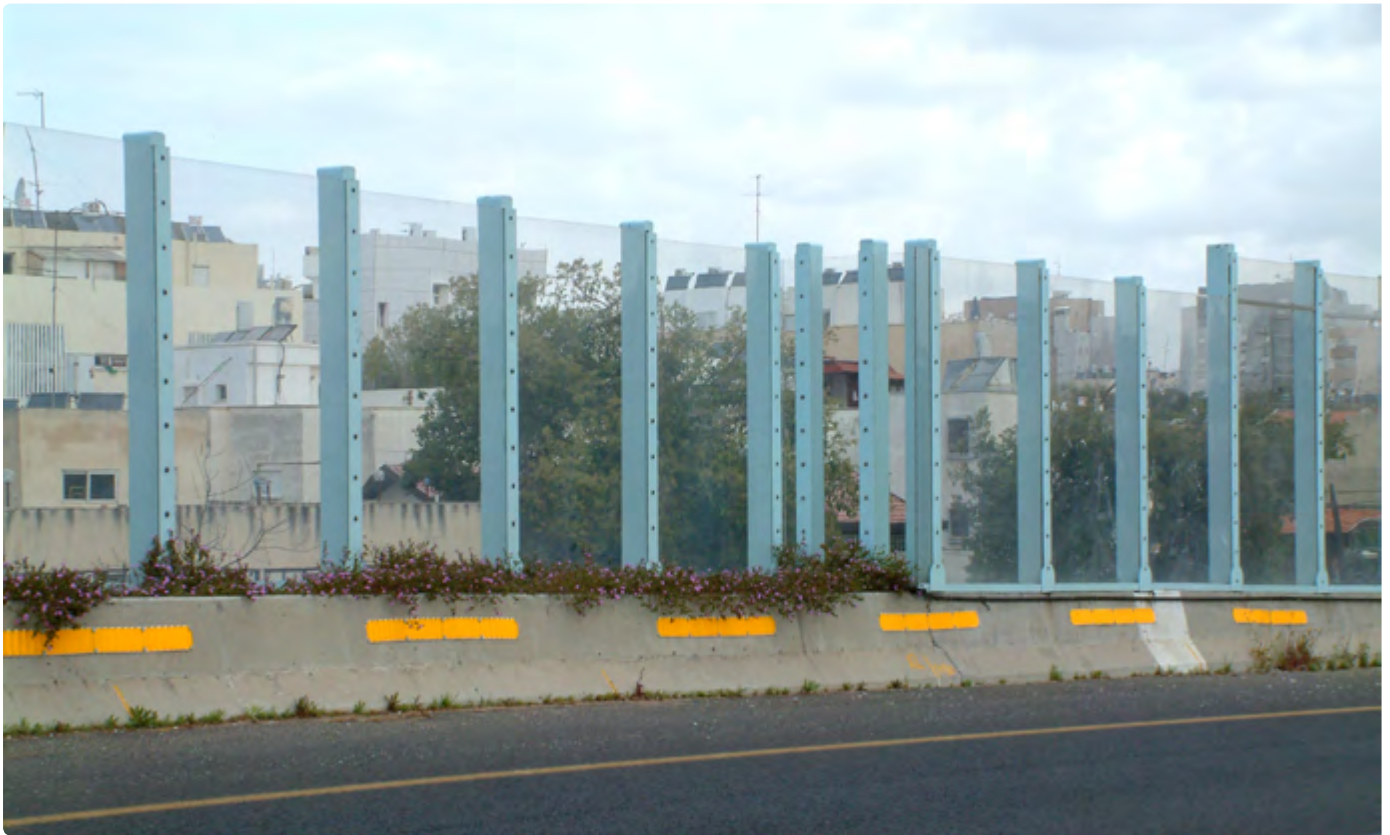
Project: Ayalon Road System - Tel Aviv, Israel (2000) | Barrier Glazing: PALGLAS® 20mm Clear
