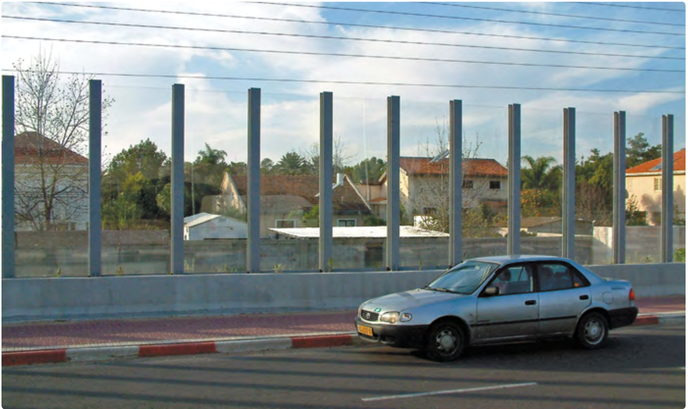
Project: Kfar Saba Interchange (Road 531) Israel (2002) | Barrier Glazing: PALGLAS® 20mm Clear
