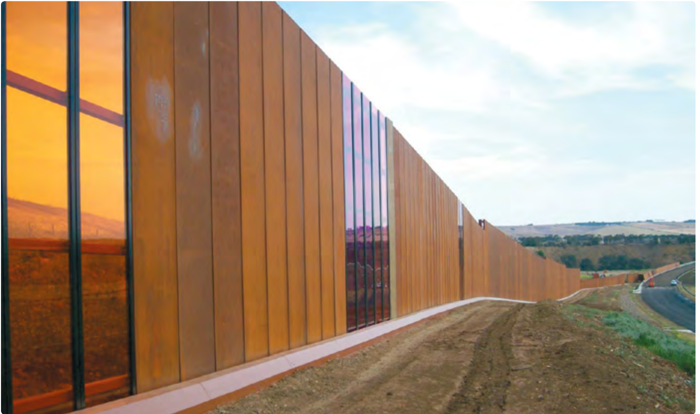
Project: Geelong Ring Road - Victoria, Australia (2008) | Barrier Glazing: PALGLAS® 20mm Custom Orange & Purple
