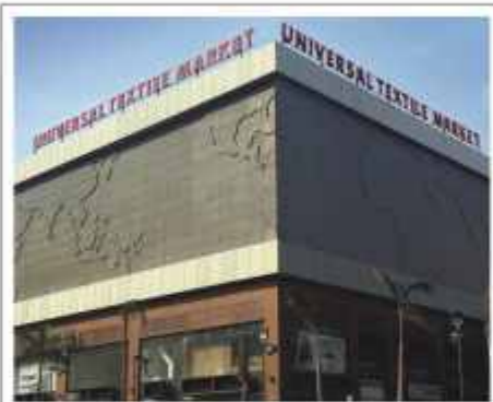
Project: Commercial Building, Surat Aspect: QUARTZ Zinc
