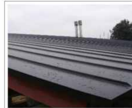
Project: Private Residence, New Delhi Aspect: ANTHRA Zinc
