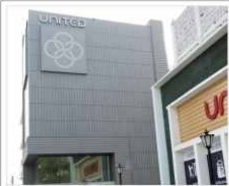
Project: Hospital, Allahabad Aspect: QUARTZ Zinc
