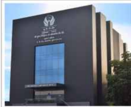
Project: Surat District Co-Operative Bank, Surat Aspect: ANTHRA Strat
