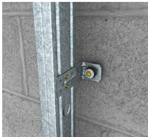
■ STDC MOUNTED ON MASONRY WALL AND SCREW FIXED TO WALL STUD
