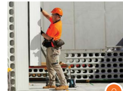
2 Panels effortlessly interlock with snap-in or slide-together mechanisms
