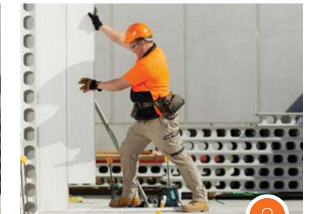
3 And simply slide down to seat into the floor tracking and form a wall
