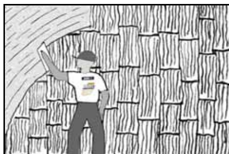
(diagram.3) smooth off and remove excess render
