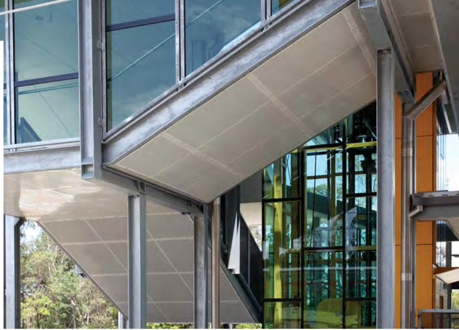
Moreton Bay Rail Link - QLD Supplied and Installed by Stoddart
