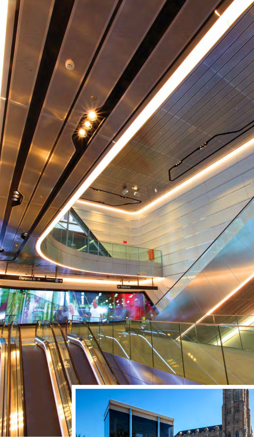
Wynyard Walk, NSW Supplied by Stoddart Custom Pattern, 3.25 Diameter Holes
