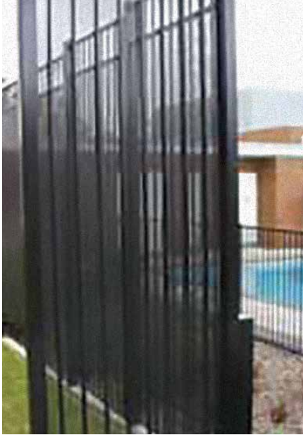
Fencing at Concord Hospital – P0648516
