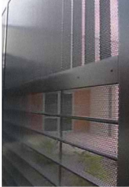
Fencing at Concord Hospital – P0648516
