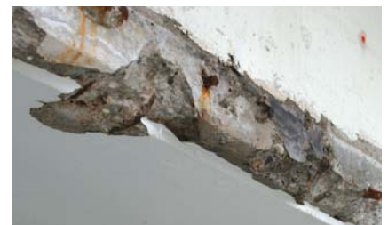
Principle 11, method 11.1 Active corrosion protection with Emaco Nanocrete AP.
