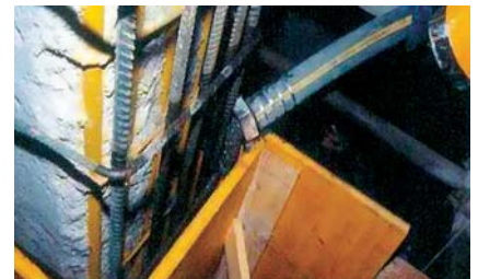
Principle 3, method 3.2 Emaco repair mortars: Emaco Nanocrete R4 Fluid recasting of elements.
