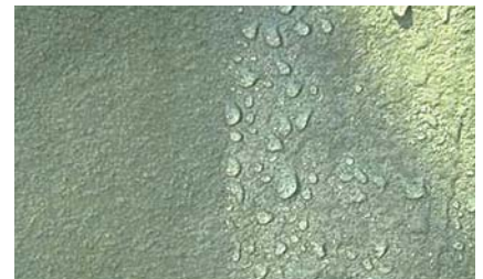
Principle 2, method 2.1 Masterseal 303 hydrophobic treatment, silane based emulsion, can be applied in many different situations or conditions.
