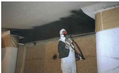
Principle 10, method 10.1 The conductive coating Emaco CP 30 cathodically protects reinforced concrete without significant additional dead load.
