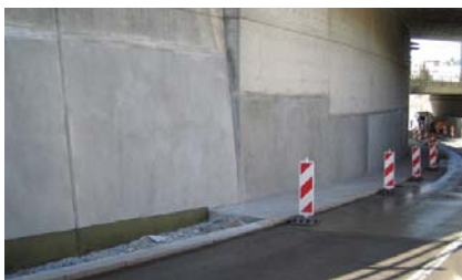
Principle 7, method 7.2 Emaco Nanocrete R4/R3 used to replace chloride contaminated concrete.
