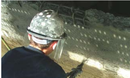
Principle 7, method 7.1 Increasing reinforcement cover with spray applied Emaco Nanocrete R4.
