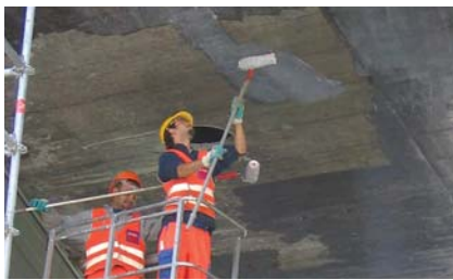
Principle 8, method 8.1 Hydrophobic treatment using Masterseal 303.
