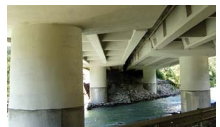
Principle 6, method 6.1 Masterseal systems: 138, 190 - epoxy / 136 - polyurethane / 185 - epoxy-cement.
