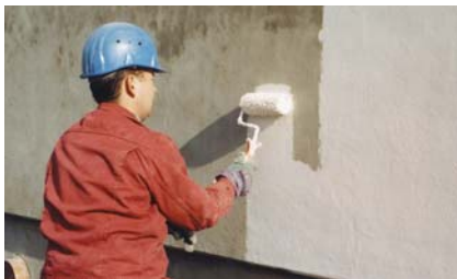
Principle 2, method 2.2 Humidity or moisture in the concrete can be controlled with Masterseal protective coatings: acrylic, EP, PU - rigid or flexible.
