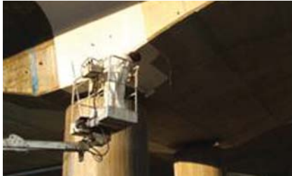
Principle 1, method 1.2 Masterseal protective coatings, available as rigid, flexible, acrylic, EP or PU materials, protect against all kinds of ingress.
