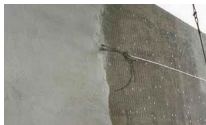
Principle 10, method 10.1 Activated titanium anodes are embedded in Emaco CP10, specially designed for optimum compatibility with the CP anode.
