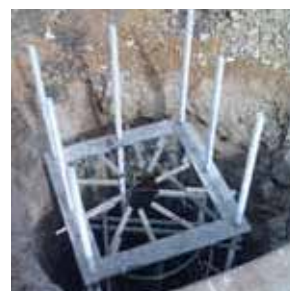
Concrete footings preparation for swing gates
