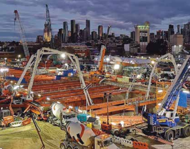
Metro Tunnel, Melbourne
