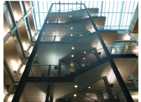
* Typical Architectural Installation
