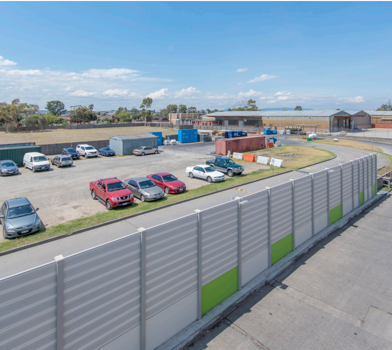
BAKERY PRODUCTION PLANT - ABSORBING WALL
