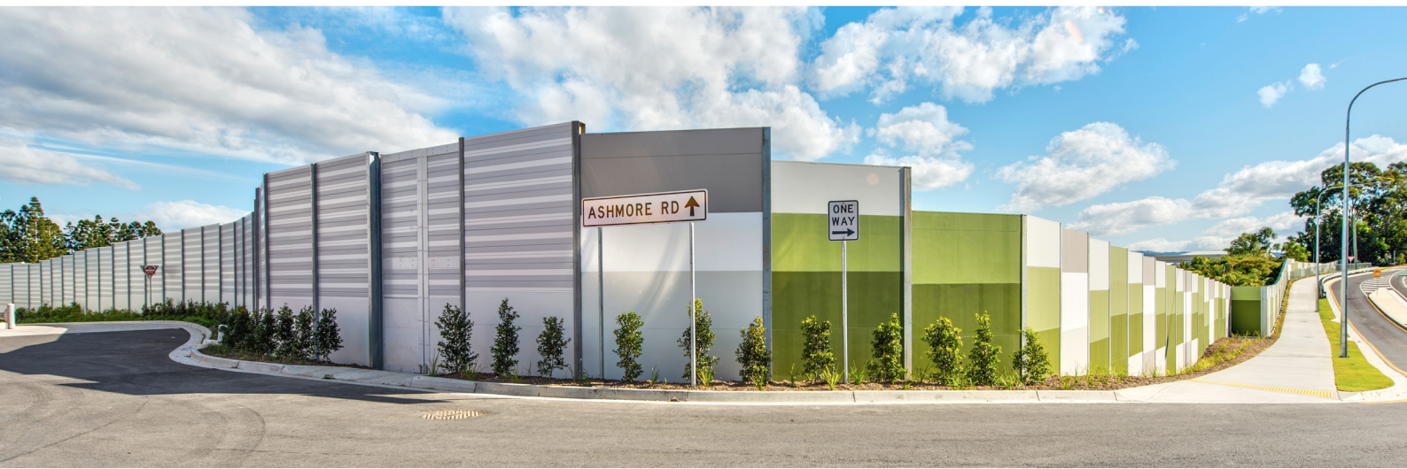
SUPERMARKET LOADING DOCK
