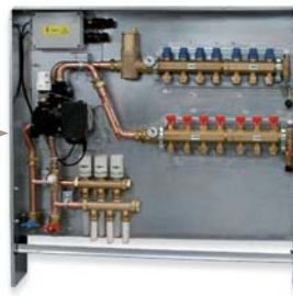
STAGE 3: installation of COMPACT mixing module/pump
