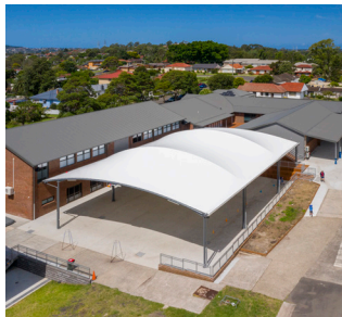
ST JOHN'S CATHOLIC PARISH SCHOOL PVC School COLA
