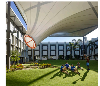
NUDGENE COLLEGE BOARDING SCHOOL PVC Custom Shade Structure
