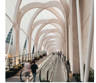
THE LINK, CHADSTONE PTFE/Gulam Pedestrian Walkway
