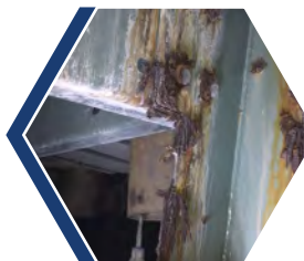
Coupling of dissimilar metals
