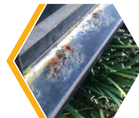
Coupling of dissimilar metals
